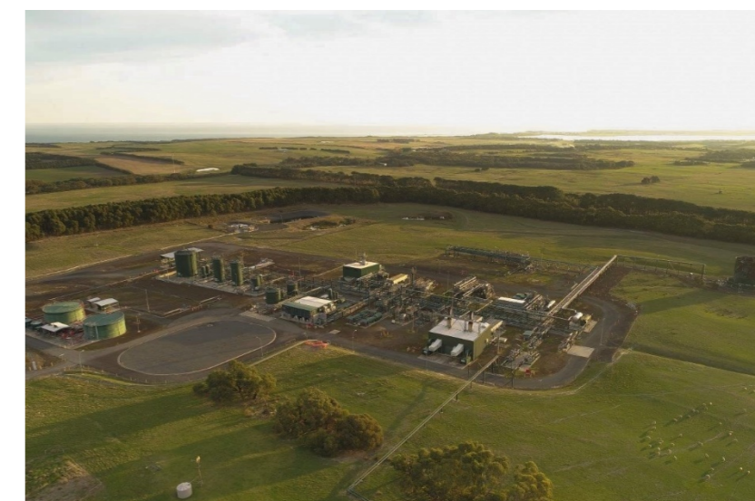
Minerva Gas Plant
