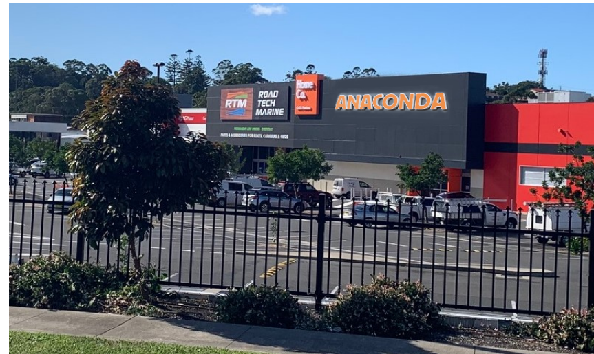
Coffs Harbour view from main road
