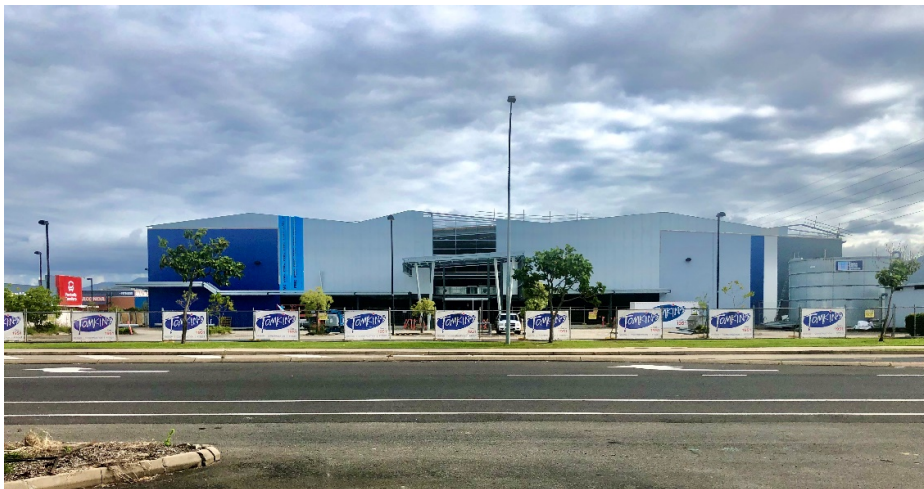
Cairns current construction as of June 2020
