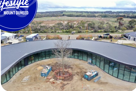
Clubhouse due for completion in September 2020
