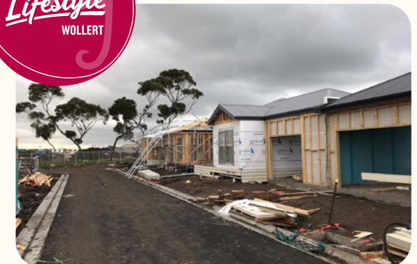
First frames underway and clubhouse under construction
