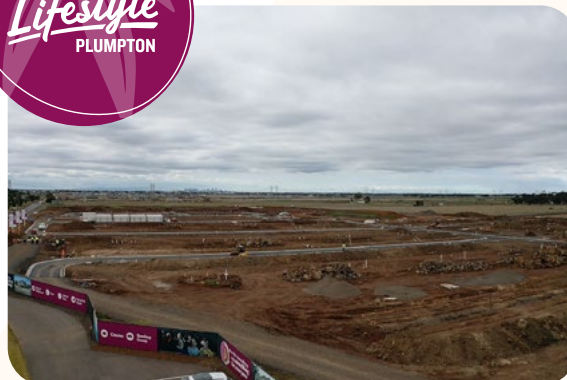
Civil works in full swing and clubhouse under construction
