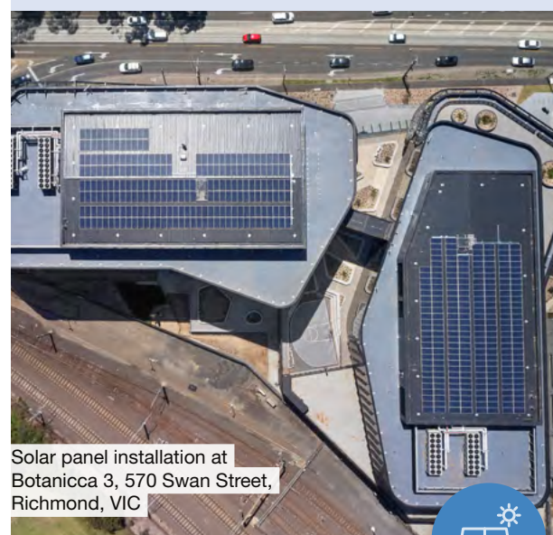
Solar panel installation at 75 Dorcas Street, South Melbourne, VIC
