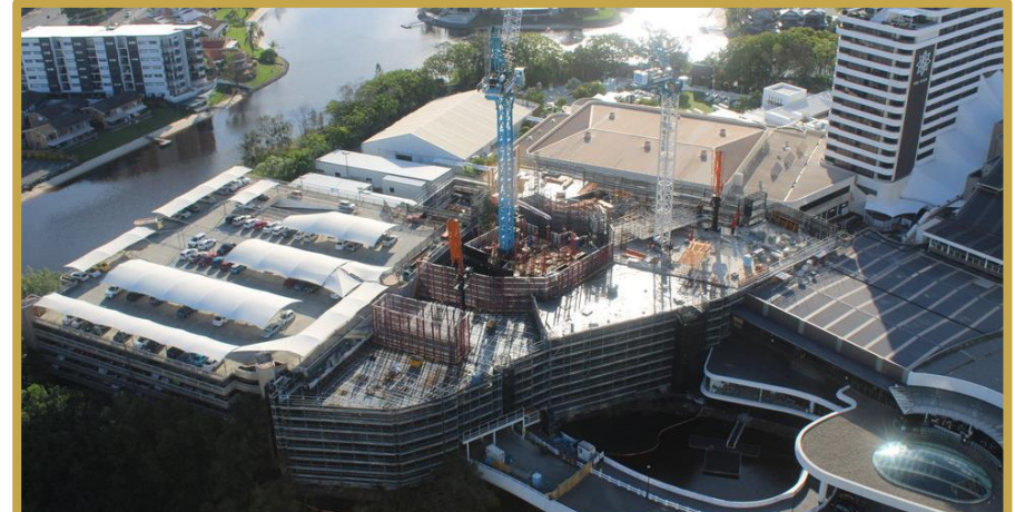
DORSETT HOTEL AND RESIDENCES (TOWER 1) FEBRUARY 2020
