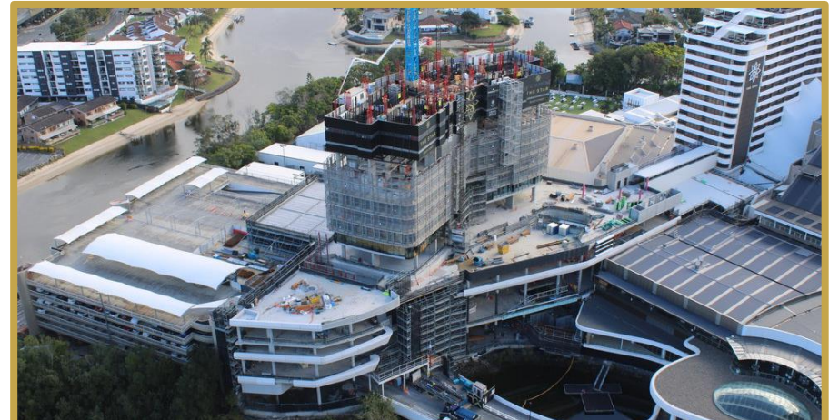
DORSETT HOTEL AND RESIDENCES (TOWER 1) AUGUST 2020
