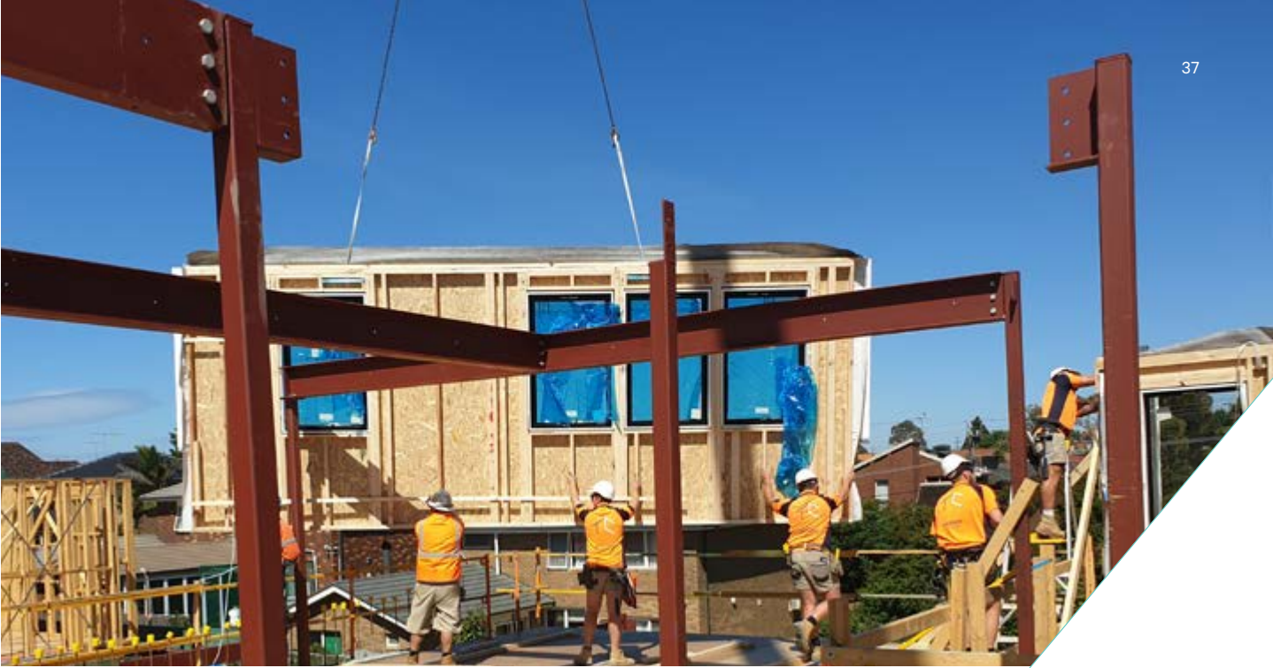
Assembling prefab homes at Tullamore, Melbourne
