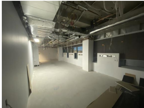
Sydney CBD: Theatre recovery construction
