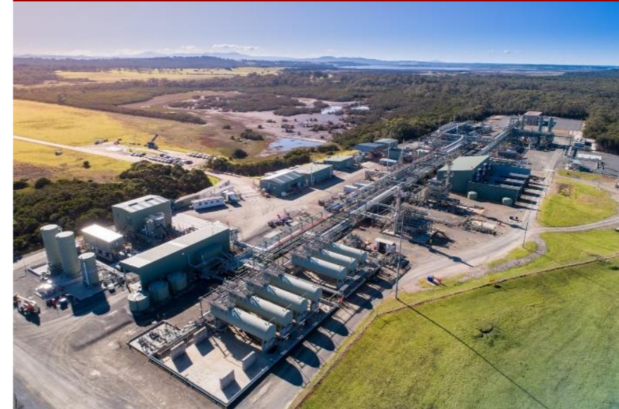
Onshore project: APA
