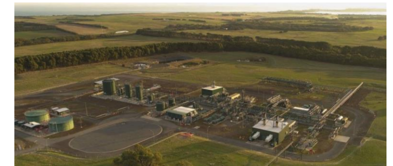
Athena Gas Plant, Onshore Otway
