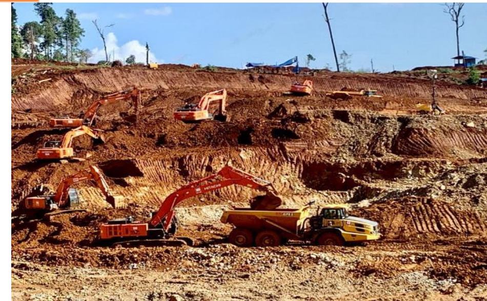
Central Pit – July 2020
