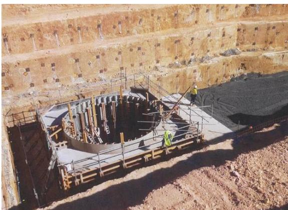
Shaft sub-brace concrete structure complete
