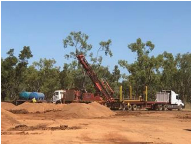
RIG UP WATER BORE DRILLING RIG
