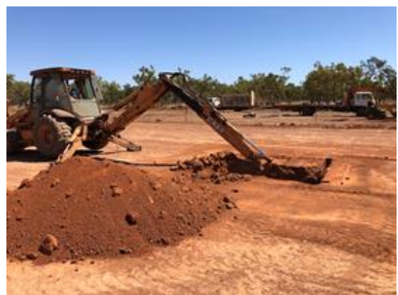
CARPENTARIA-1 WELL CELLAR BOX EXCAVATION
