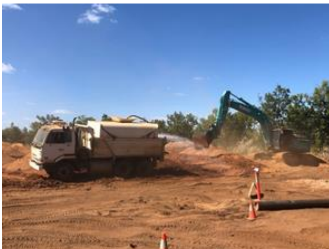
CONDITIONING/SHAPING BUNDS AROUND THE CARPENTARIA-1 WELL SITE
