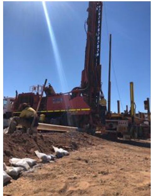
DRILLING IMPACT MONITORING BORE
