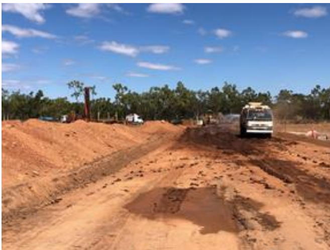
CARPENTARIA-1 WELL PAD PREPARATION
