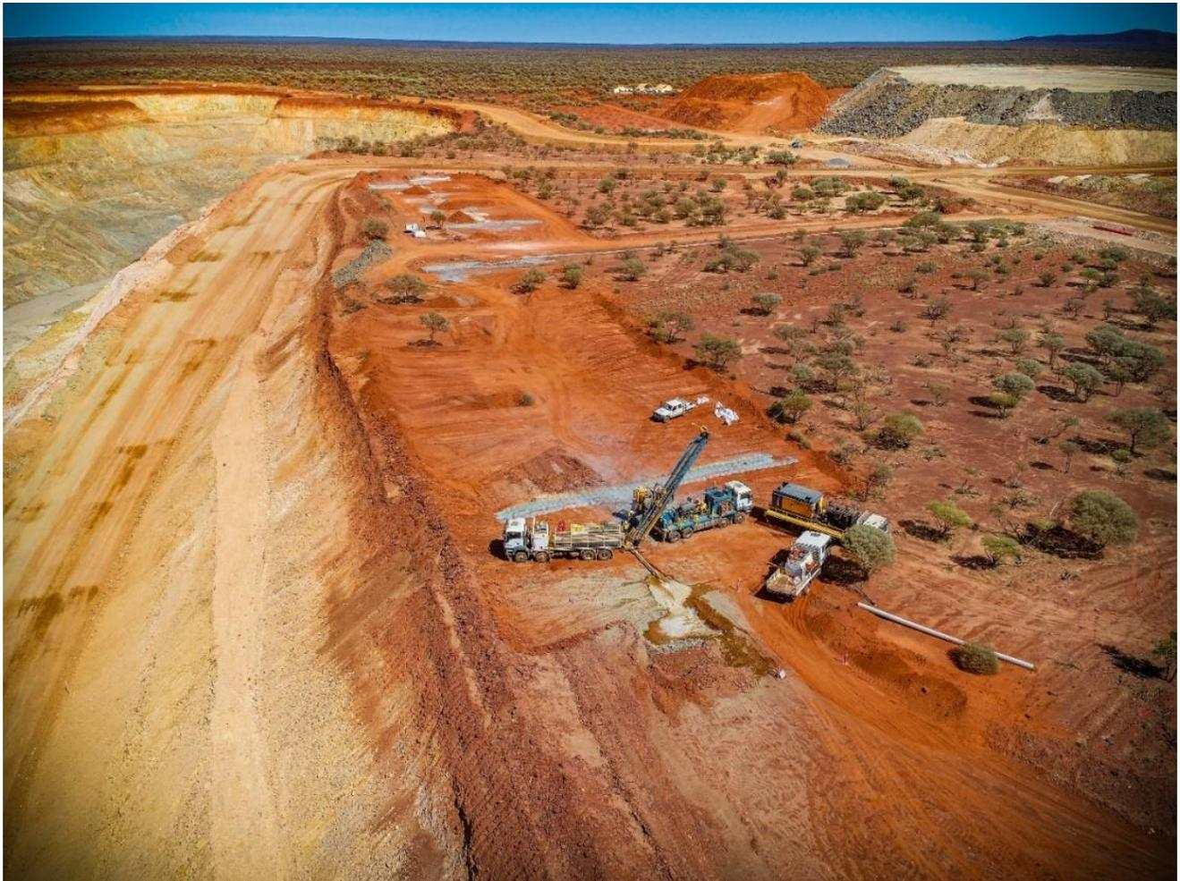
**Figure 2:** Aerial photograph of drill rig drilling DGRC0582 (40m @ 1.3g/t Au) at Gilbey's, Dalgaranga (looking south)
