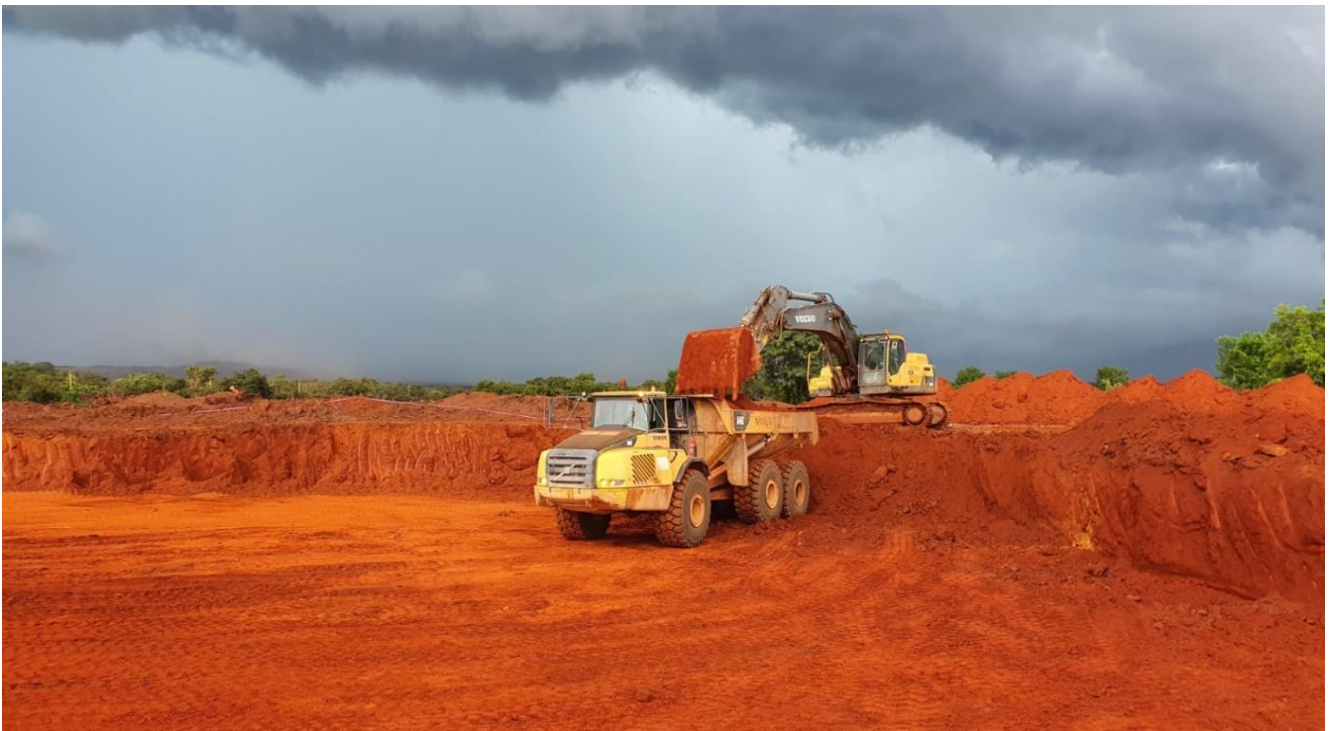
Figure 1: Establishment works at the Cashew mining operation
