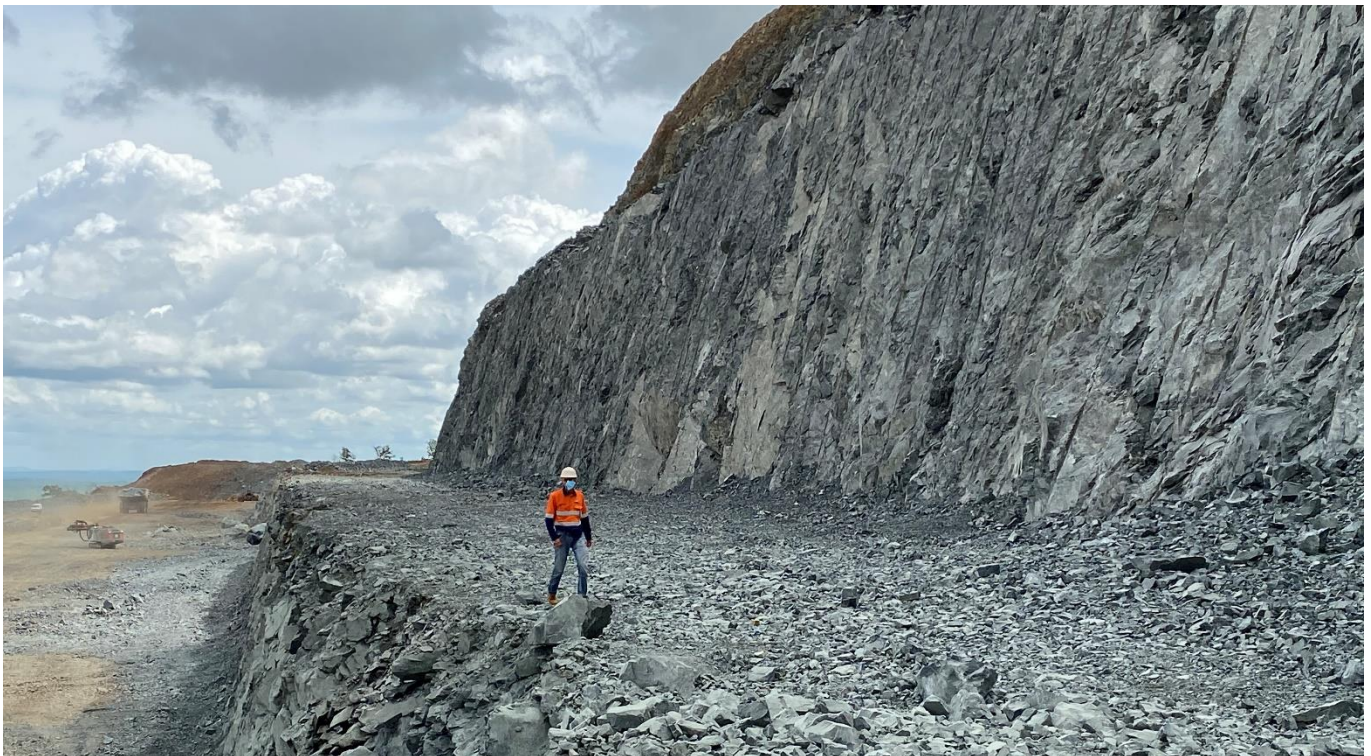
Figure 2: Open pit operations at Mako
