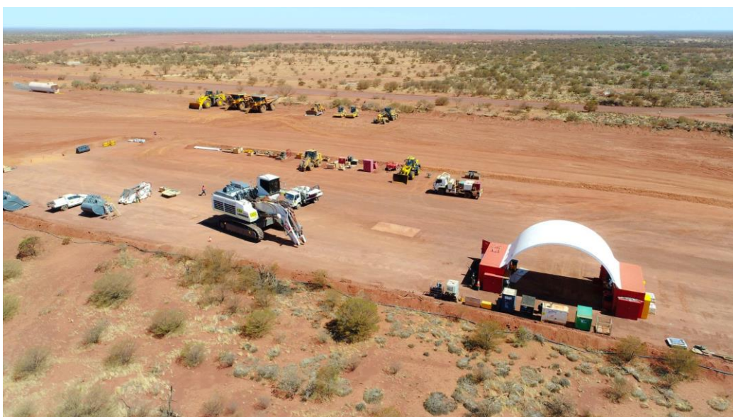
Mobilisation of mining contractor
