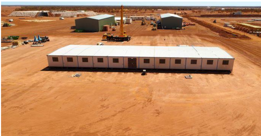
Administration office, Maintenance workshop and stores shed
