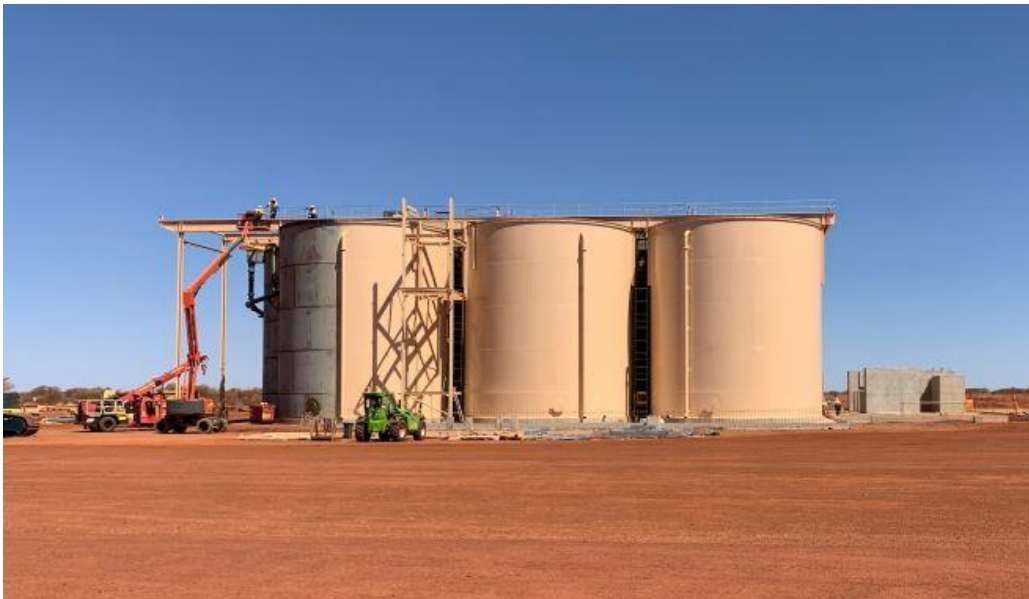
CIL tank steelwork and painting
