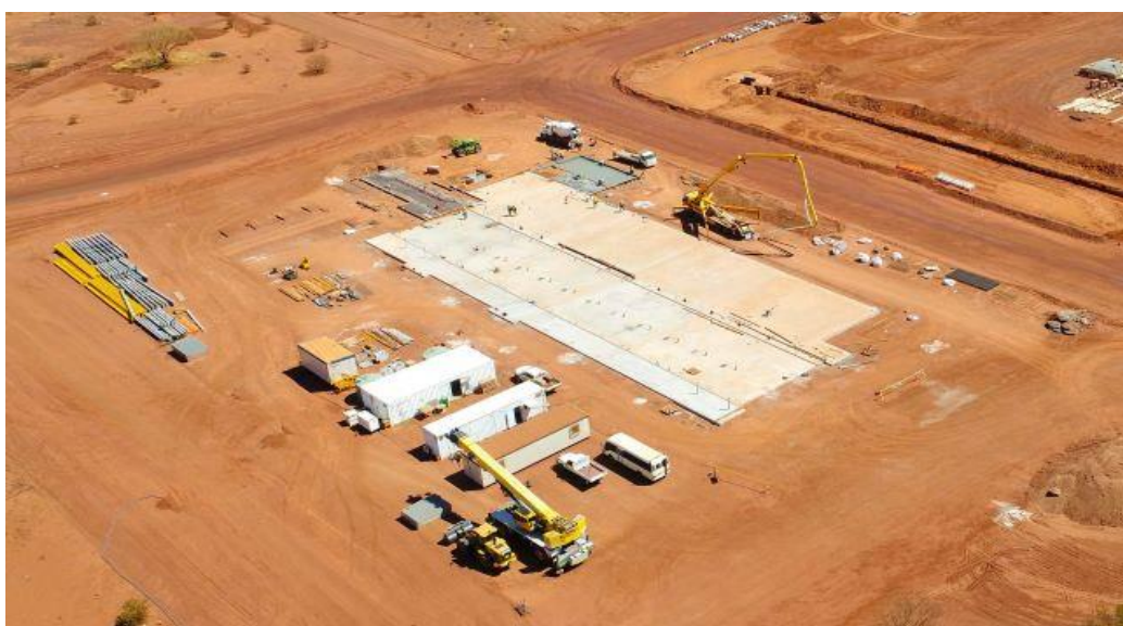
Foundations for power station
