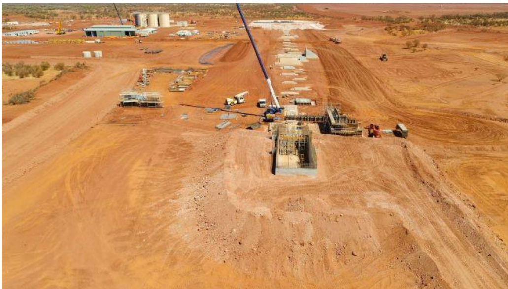
Foundations for crushing circuit
