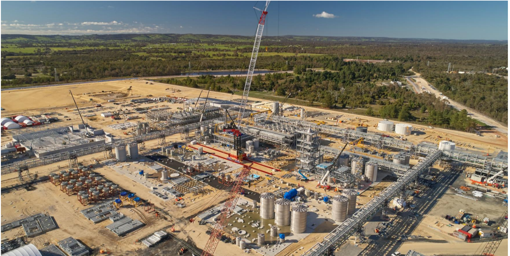
Construction underway at the MARBL Lithium Joint Venture's Kemerton Plant, south-west region, WA.
