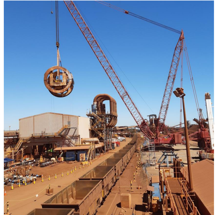
BHP's Nelson Point, Pilbara region, WA.
