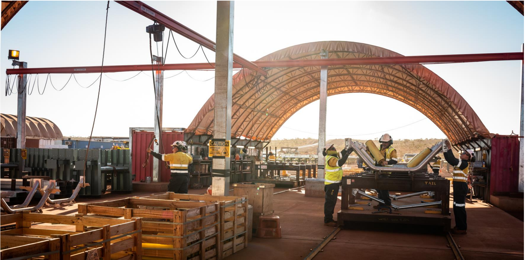
Conveyor module assembly at BHP's South Flank Project, Newman, WA.
