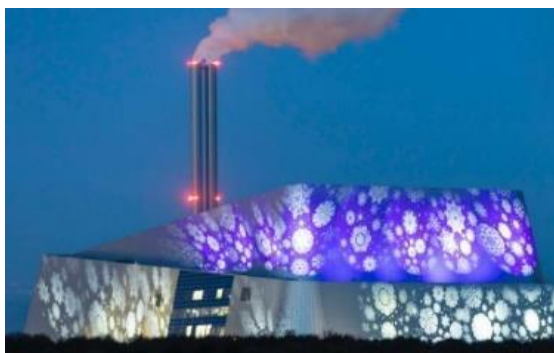
Covanta, Dublin, energy-from-waste
