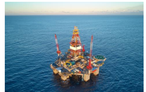
Drilling of Sole-3
