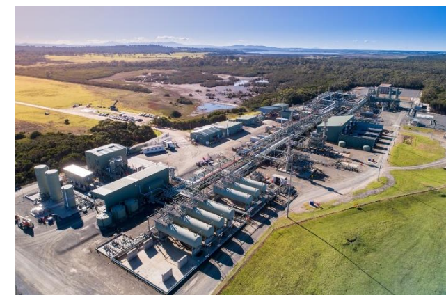
Orbost Gas Processing Plant
