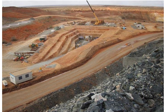
Shaft winder house foundations and raise bore rig (at top right)
