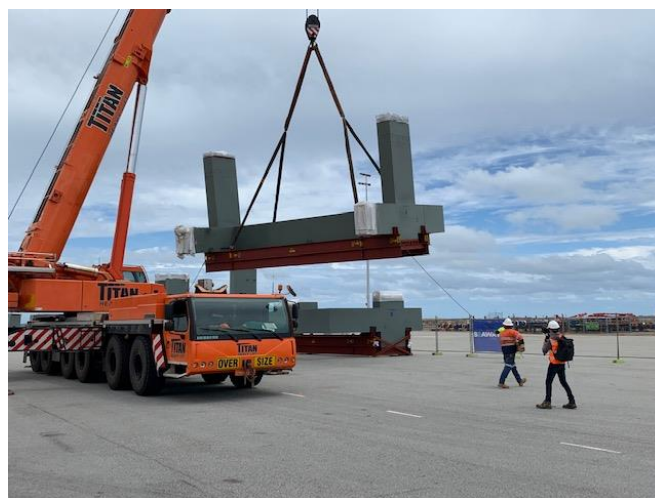
Shaft headframe sections being offloaded
