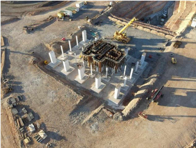
Shaft winder house foundations and raise bore rig (at top right)
