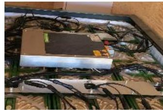
30 kW scalable salt-water battery technology at Touquoy site, powered by solar panels
