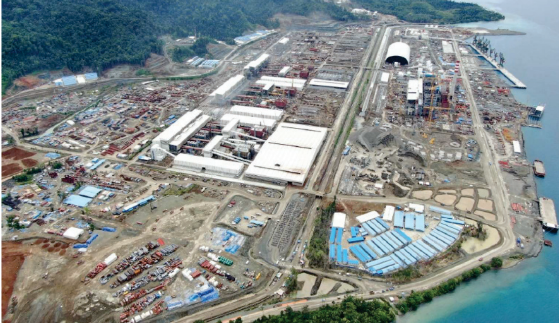
Nickel Mines – IWIP aerial photo
