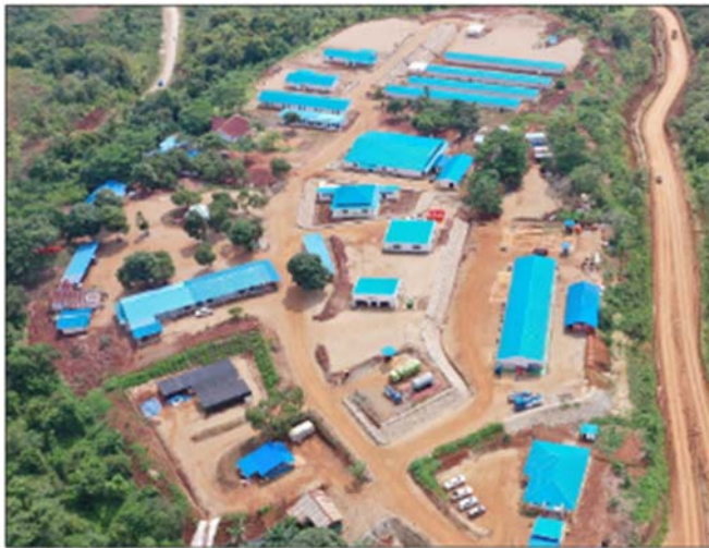
Accommodation, technical offices, CSR office and training facilities
