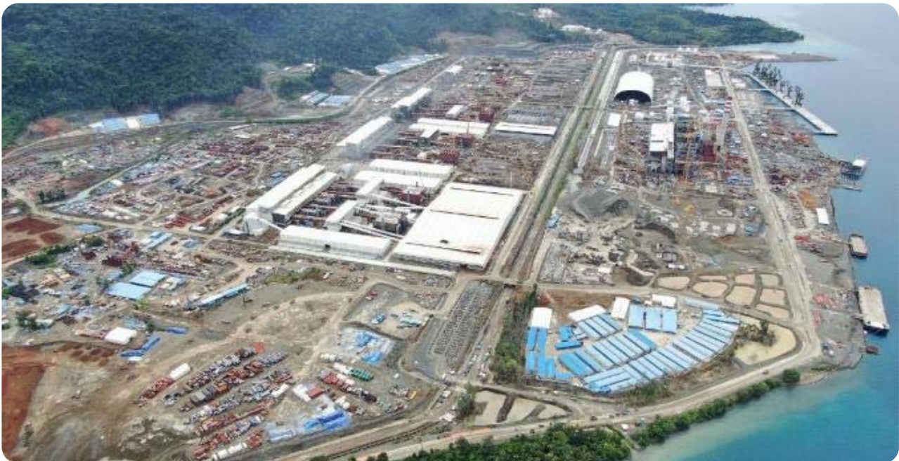
Aerial photo of the IWIP
