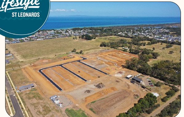
Land settled in July 2020. Civils program well progressed. Clubhouse construction commenced.
