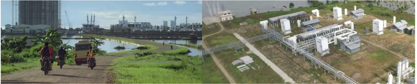
The Sengkang LNG Plant has a design capacity of 2 mtpa, consisting of 4 modular 500,000 tpa trains, an import/export and jetty facilities.
