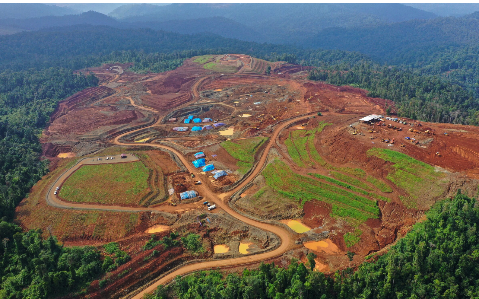
Aerial view of the Bete Bete pit at the Hengjaya Mine.
