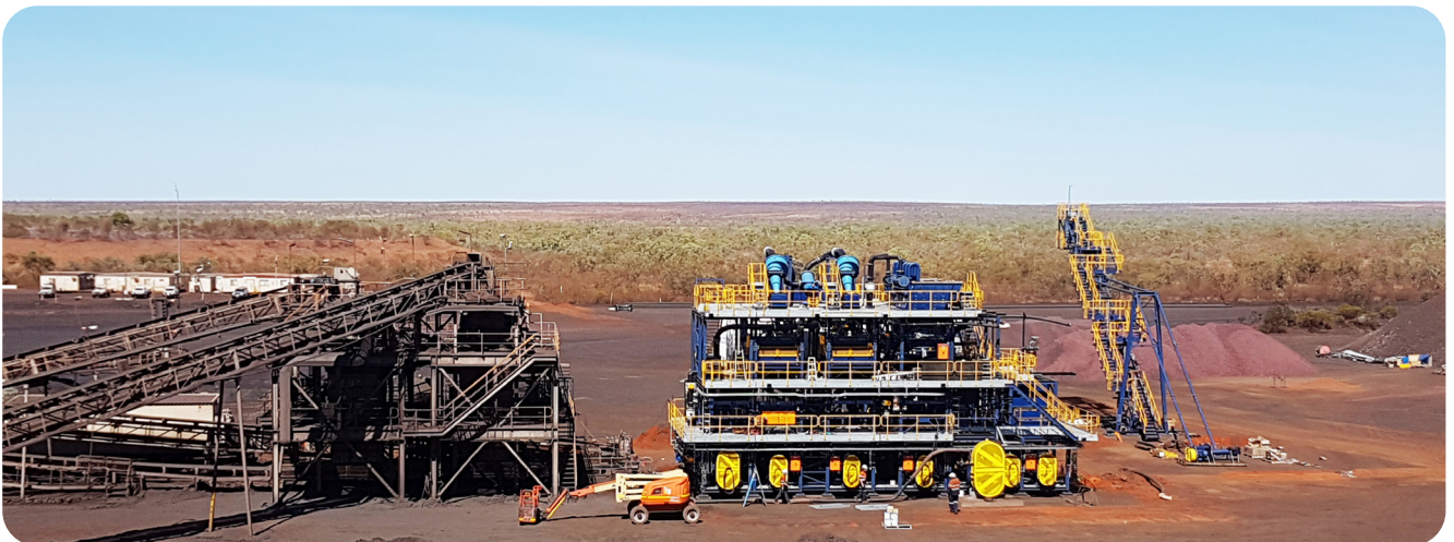
Figure 2. Ultra-Fines Processing Facility
