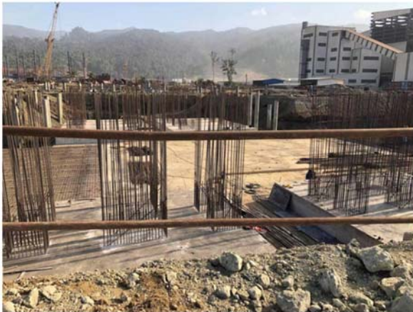
Foundations for lines #1 and #2
