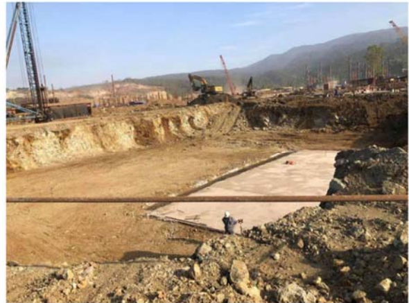
Foundations for lines #3 and #4
