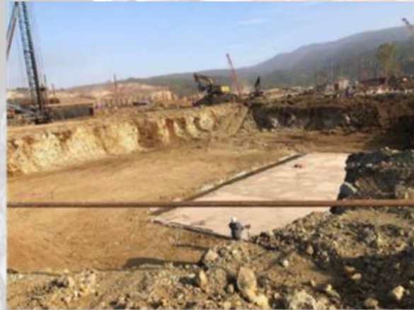
Foundations for Lines #3 and #4
