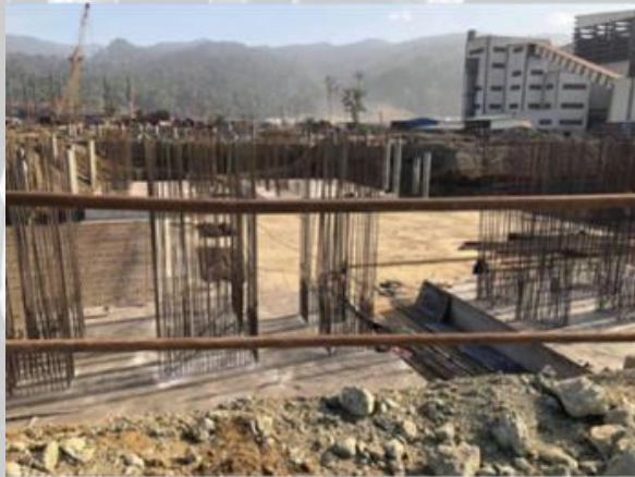
Foundations for Lines #1 and #2
