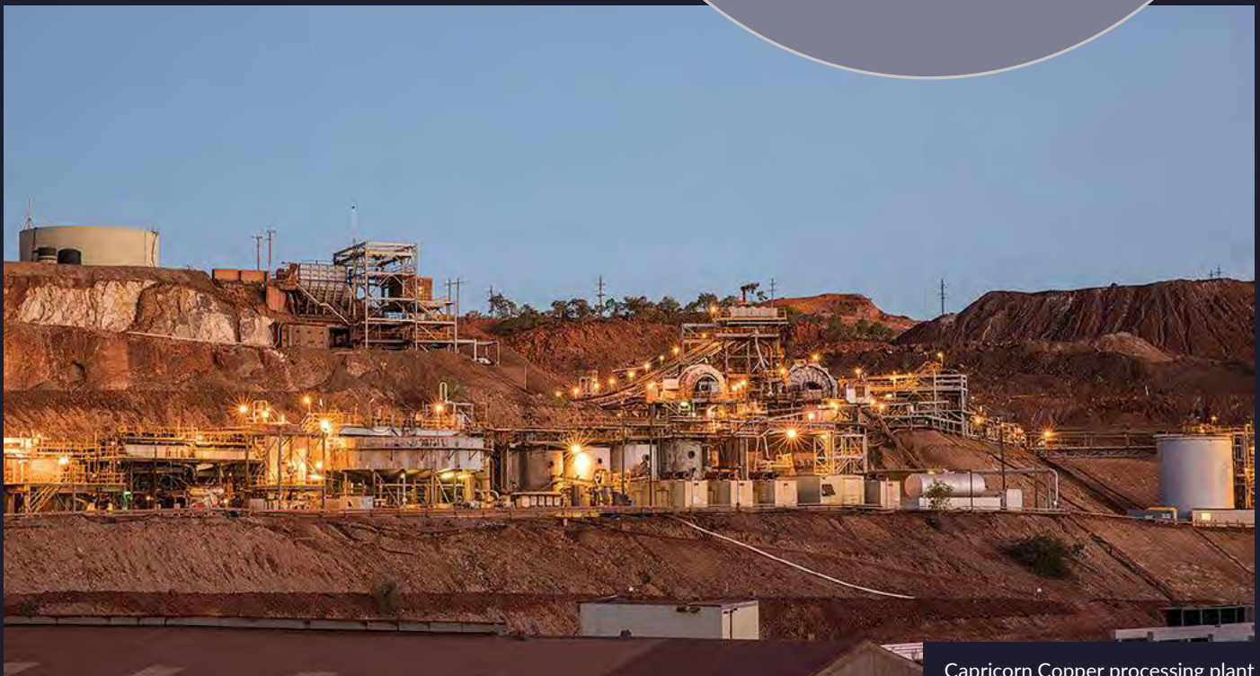
Capricorn Copper processing plant
