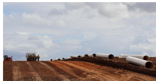
Land preparation and irrigation system installation, central Qld, May 2021.
