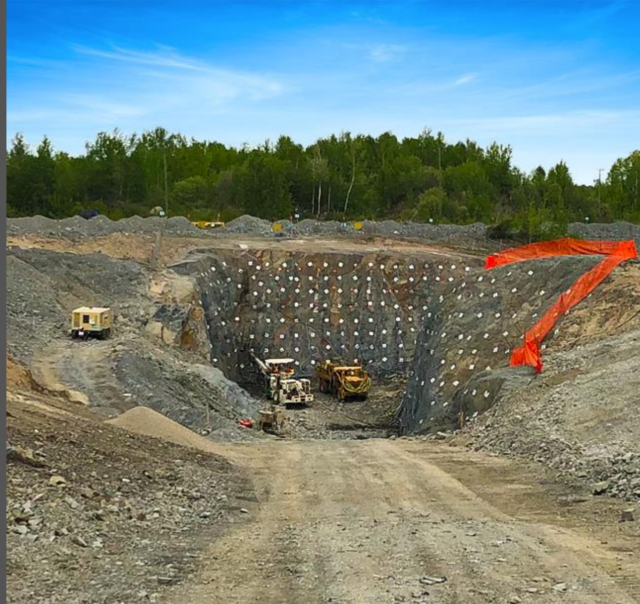
Campbell Young Dickenson box cut construction commenced in the March 2021 quarter
