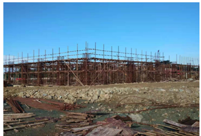
Column reinforcement for Electrostatic Precipitator
