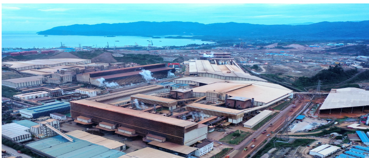
Hengjaya and Ranger RKEF operations
