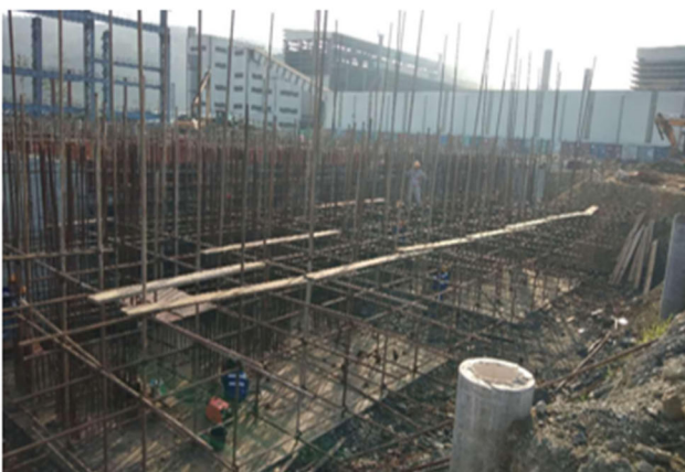
Scaffolding support for the RKEF Lines
