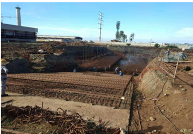
Foundations for Dry Ore shed
