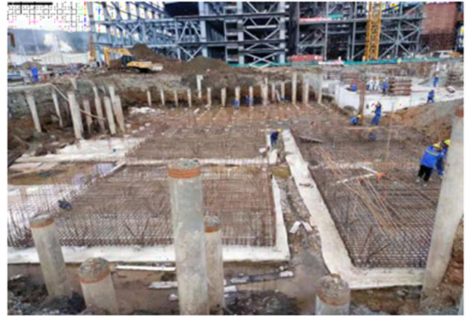
Foundations for ANI powerplant
