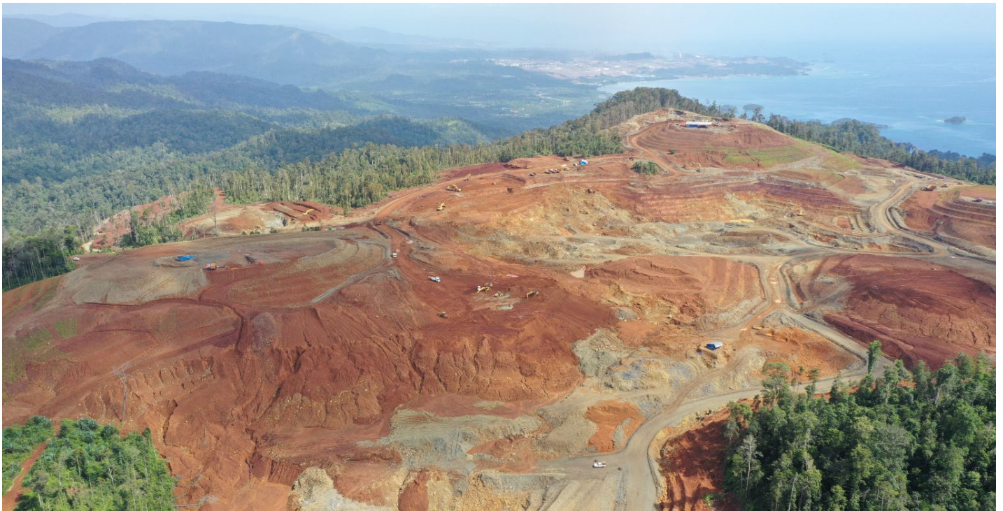
Bete Bete pit operations (foreground right is east expansion area with IMIP in the background)
