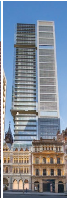
Olderfleet, 477 Collins Street MEL
