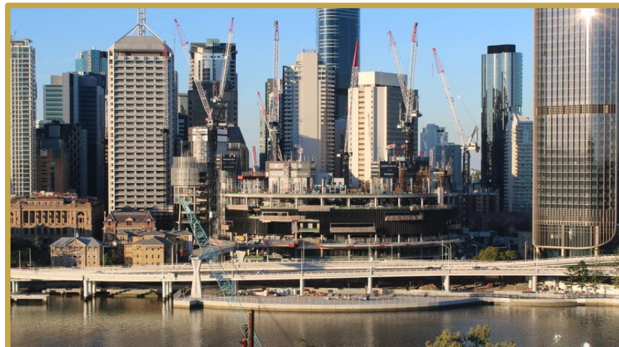
VIEW FROM SOUTH BANK – AUGUST 2021
