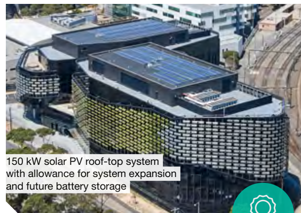
Botanicca 3, Richmond, VIC – building facade features a state-of-the-art curtain wall fitted with perforated sunshades
