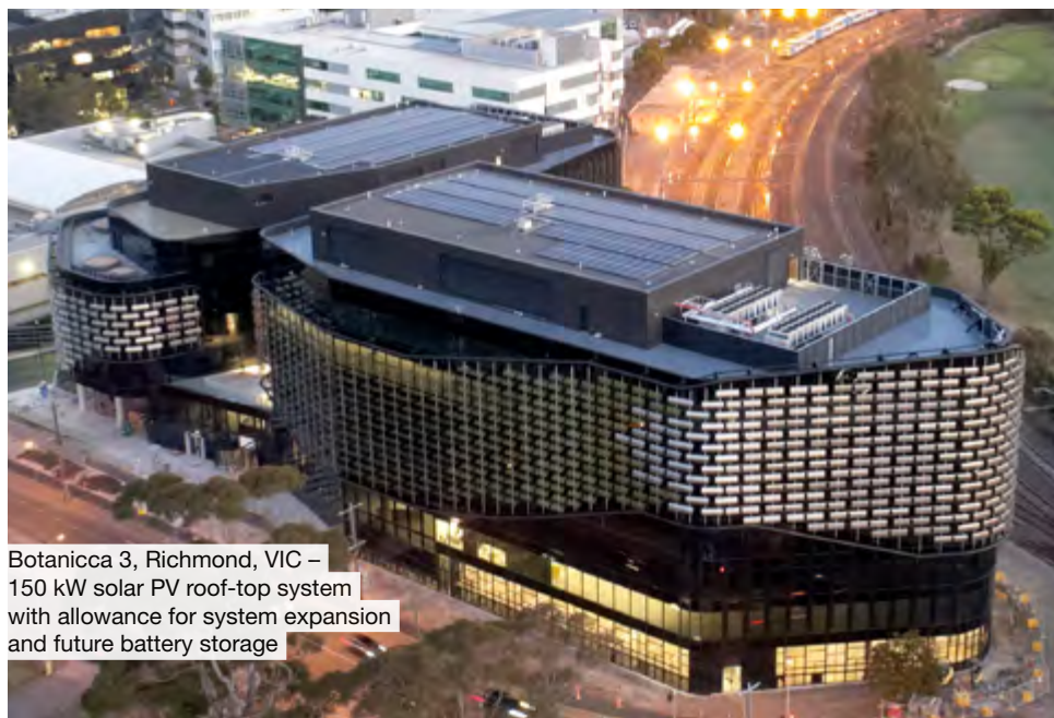
3 and 5 Murray Rose Avenue, Sydney Olympic Park, NSW – 100 kW and 130 kW roof-top solar PV systems, respectively
