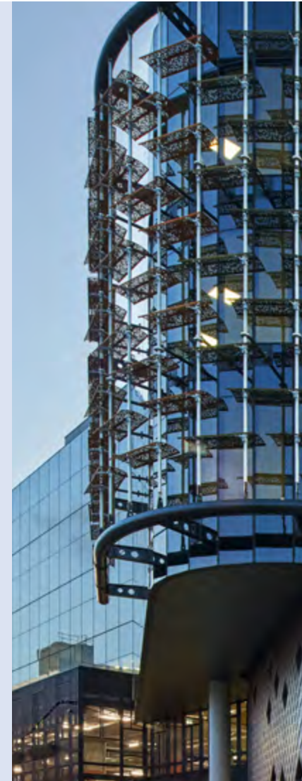
Botanicca 3, Richmond, VIC – building facade features a state-of-the-art curtain wall fitted with perforated sunshades which enhance energy efficiency
