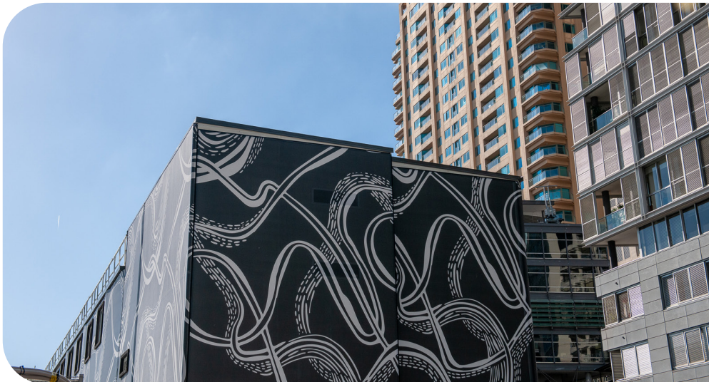
Lendlease Administration Building, New South Wales
