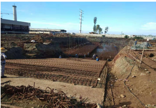
Foundations for Dry Ore shed
