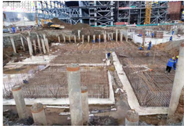
Foundations for ANI powerplant
