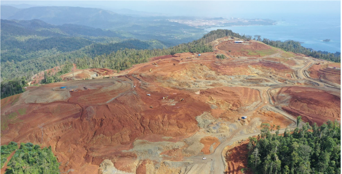
Bete Bete pit operations (foreground right is east expansion area with the IMIP in the background)
