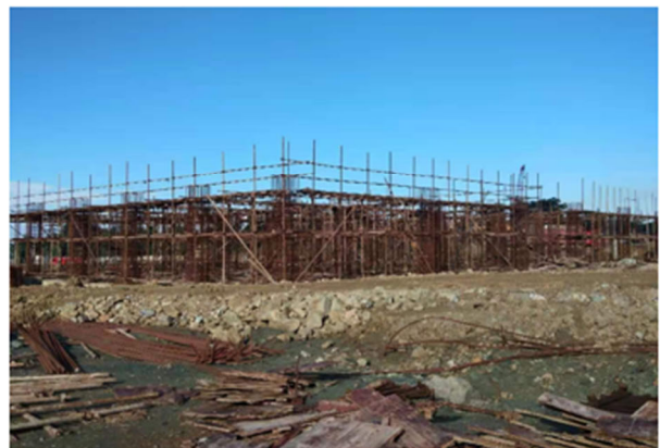
Column reinforcement for Electrostatic Precipitator
