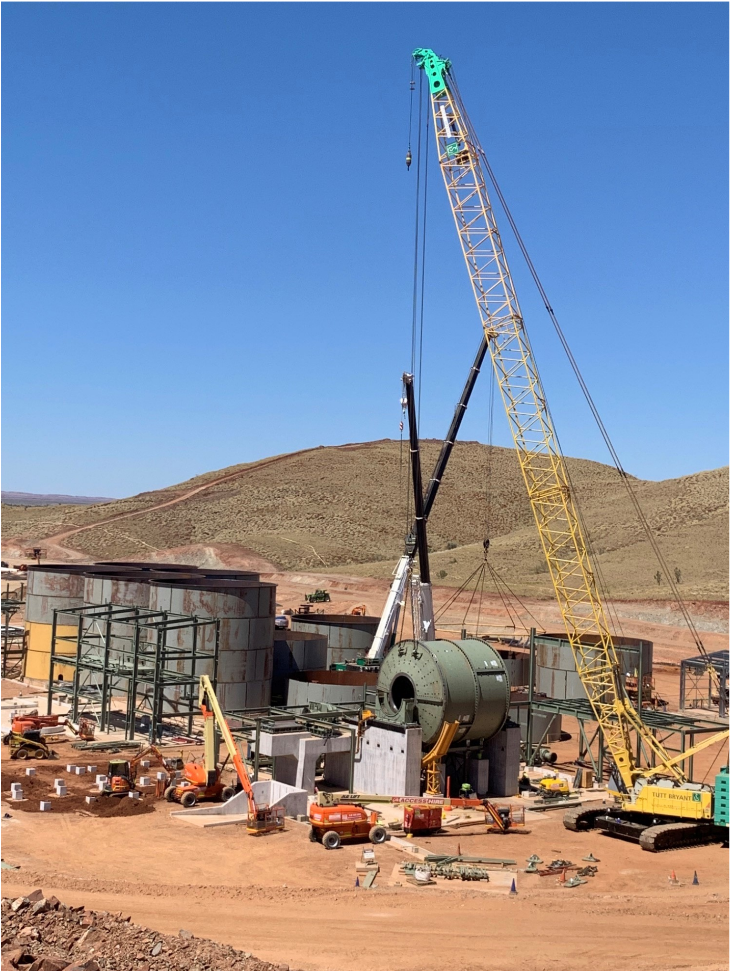
Figure 3: Mill Installation
