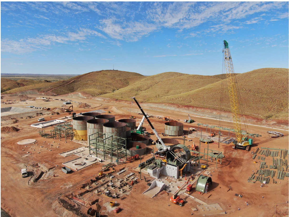
Figure 2: Mill and Tank Area
