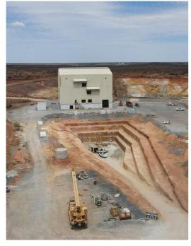
Raise bore machine site and winder house construction
