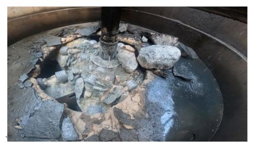
The raise bore head breaking through at surface
