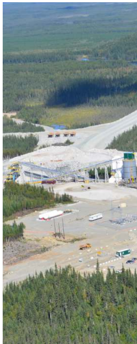
North American Lithium operation
