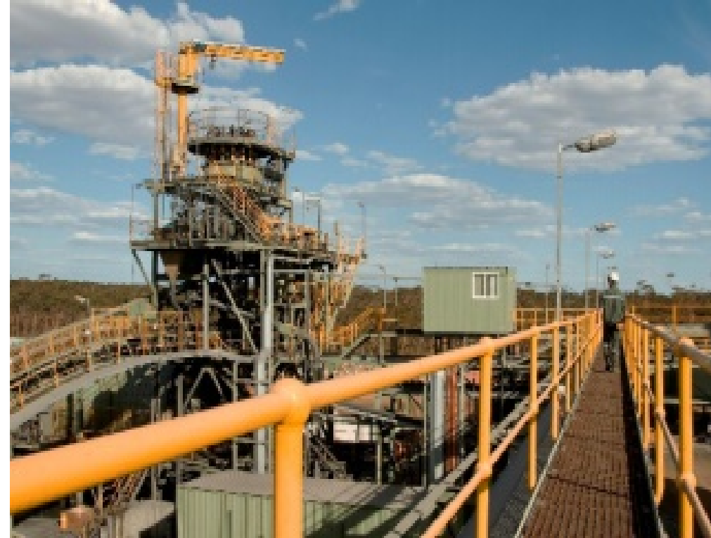
Lake Johnston processing plant
