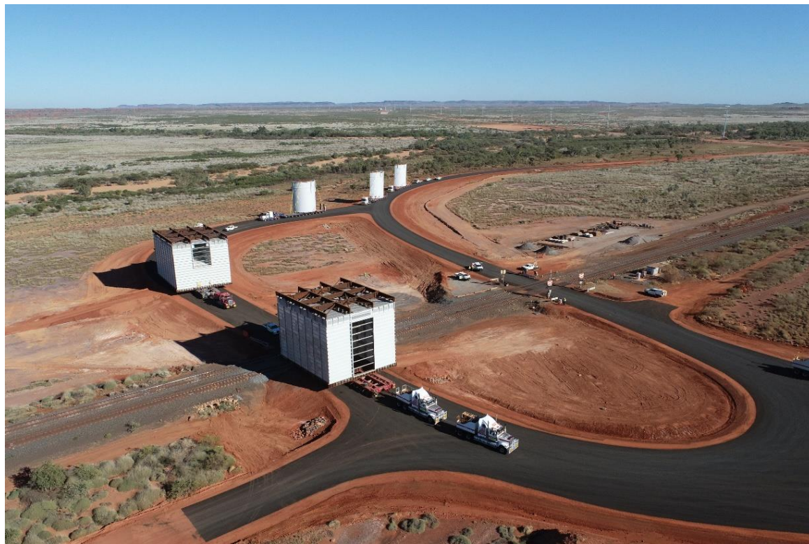
Delivery of large modules to Iron Bridge
