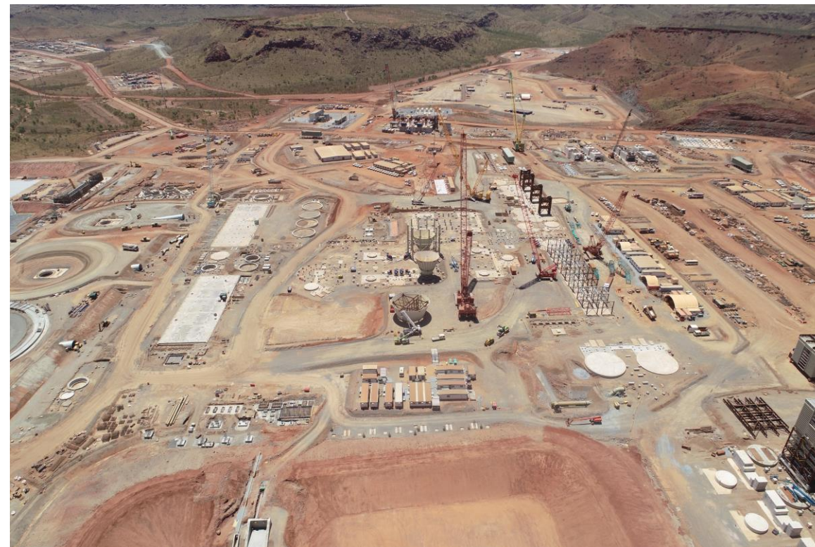
Construction of the ore processing facility
