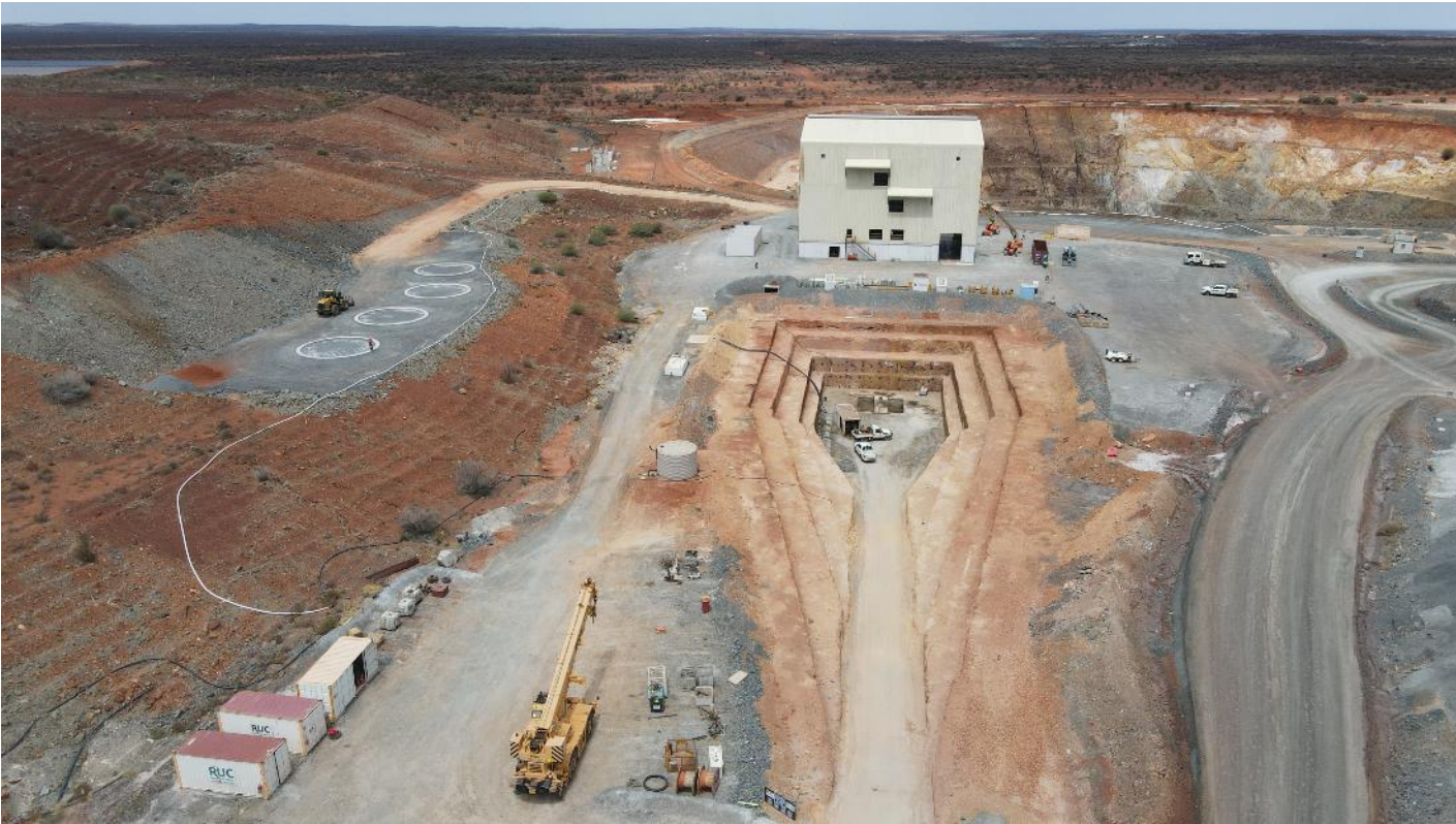
Winder house complete ready for winder installation
