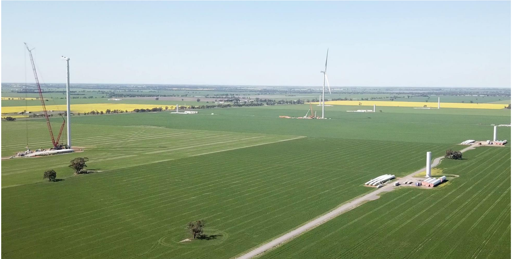
Murra Warra Stage 2 balance of plant works underway, regional Victoria.
