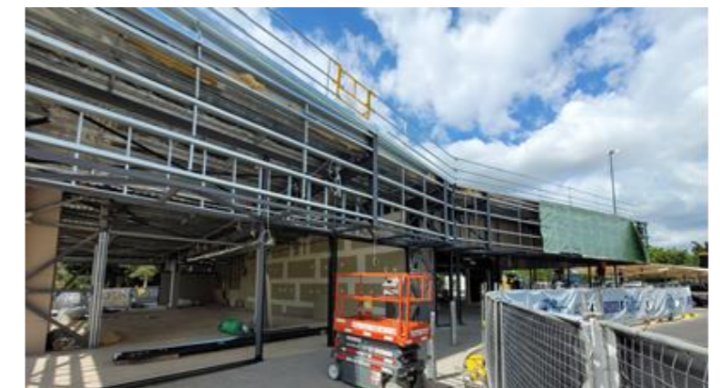
SPRINGFIELD FAIR – 600SQM PAD-SITE CONSTRUCTION UNDERWAY
