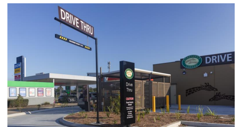
BALLINA CENTRAL 50% MILESTONE ACHIEVED WITH ZARRAFFAS COMPLETED
