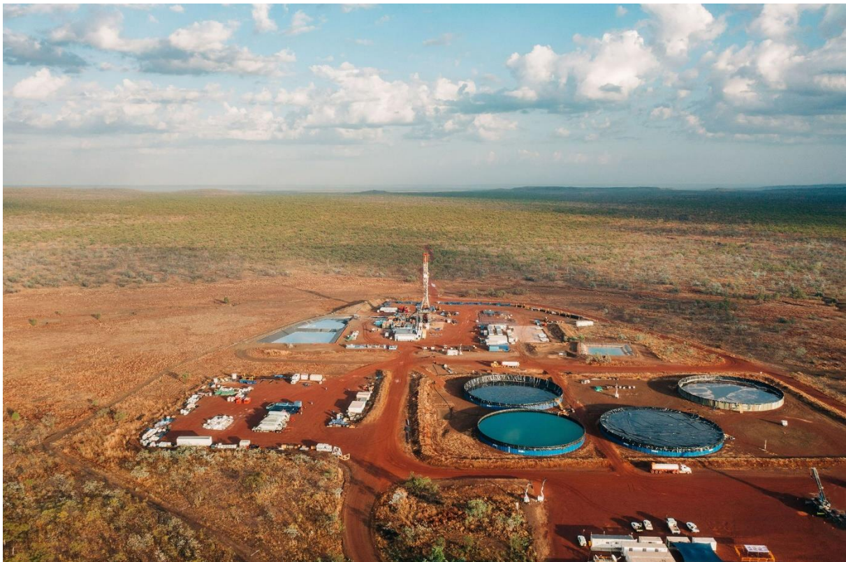
Figure 1: Drilling operations completing in EP 161, November 2021
