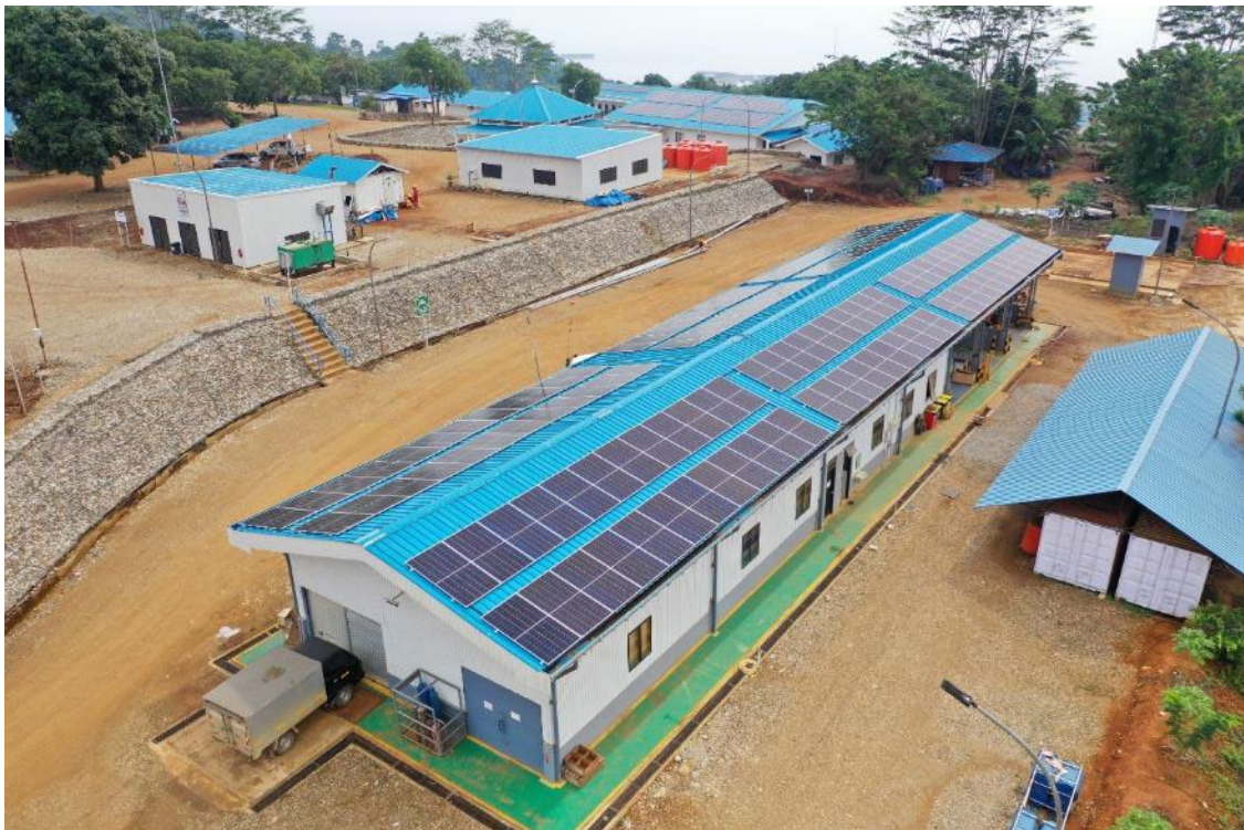
450kWp solar panel installation at the Hengjaya Mine camp
