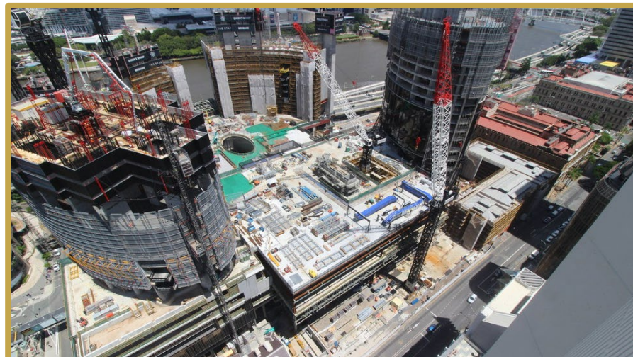
VIEW FROM GEORGE STREET – FEBRUARY 2022
