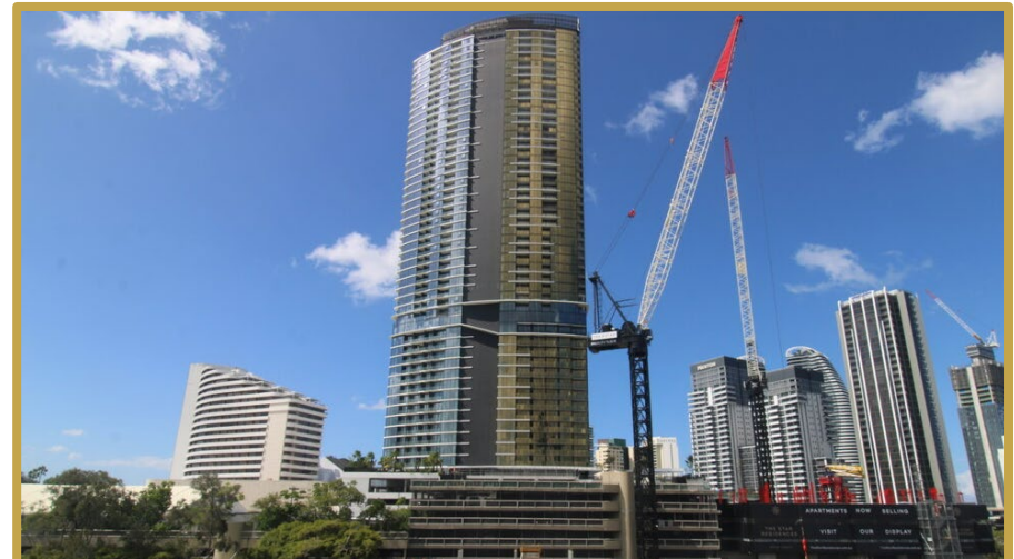
TOWER 2 CONSTRUCTION – FEBRUARY 2022
