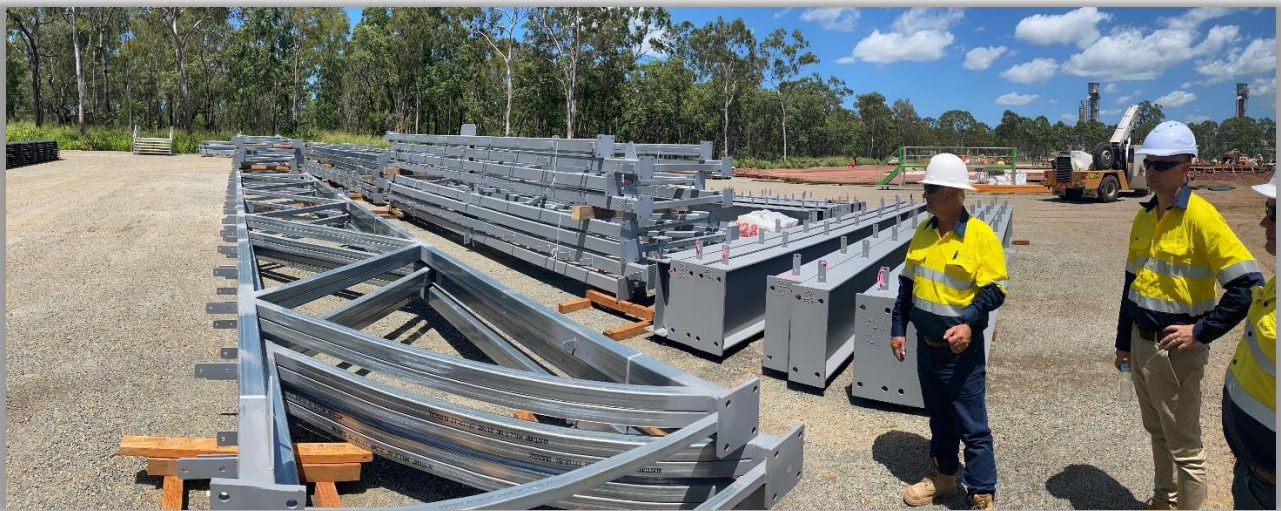
Main PPF building steel delivered on site, ready for erection
