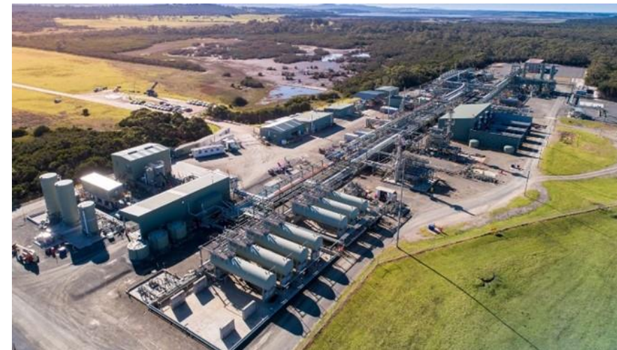
Orbest Gas Processing Plant, owned and operated by APA
