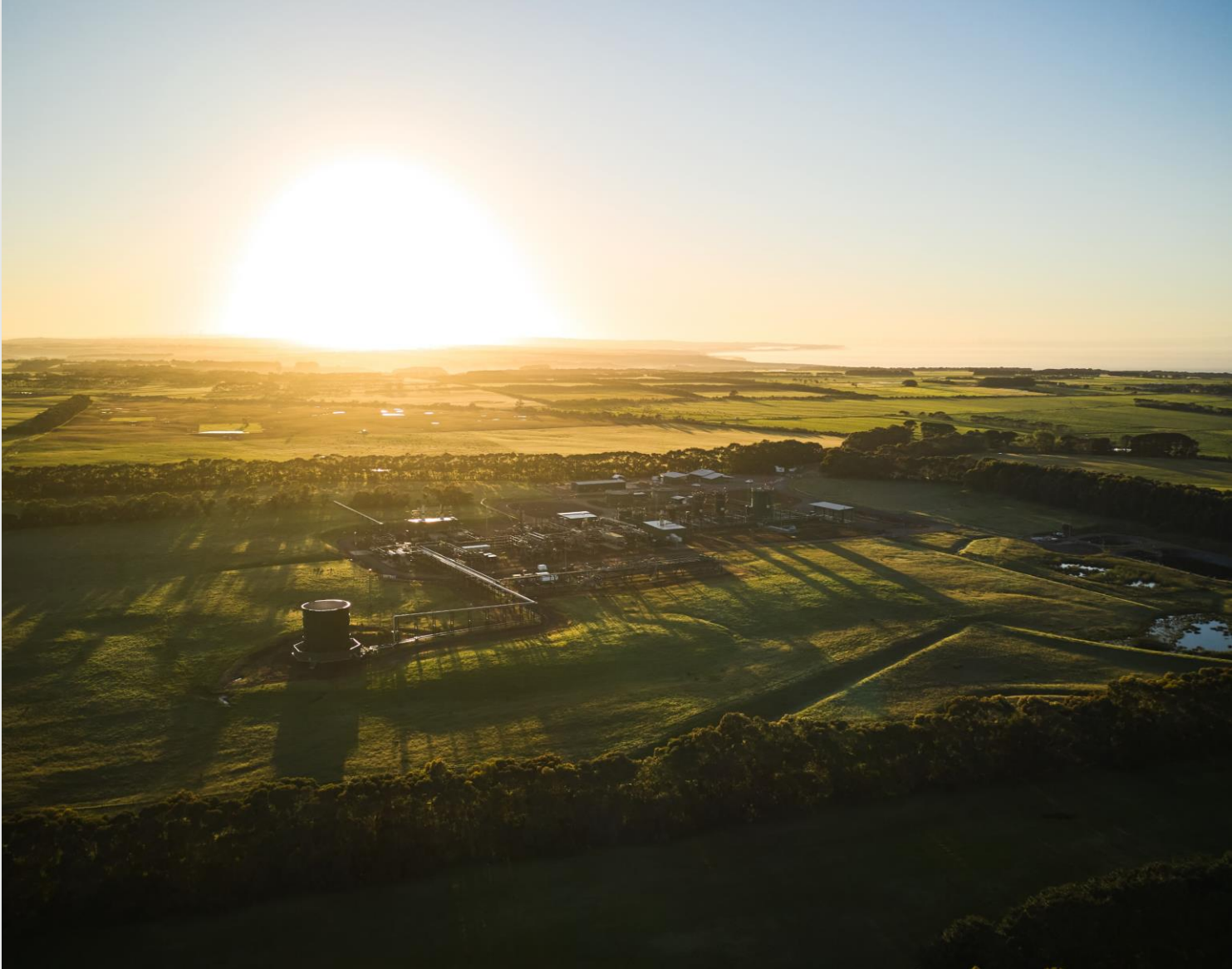
Athena Gas Plant
