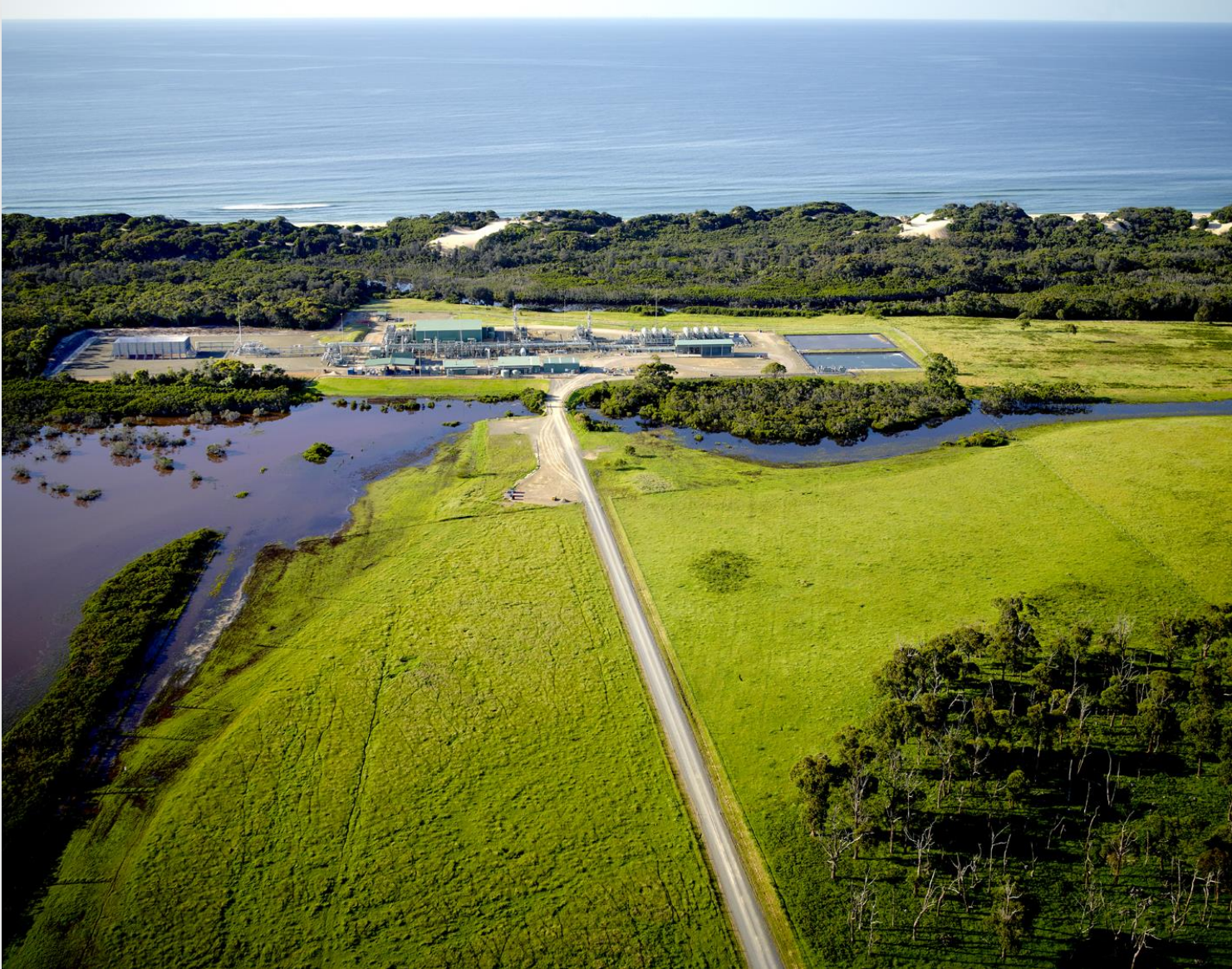
Orbost Gas Processing Plant
